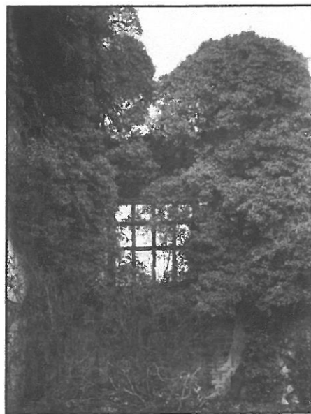
Houghton House ruins before conservation.
